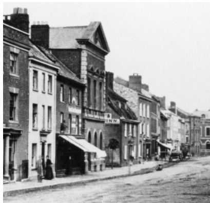
Two photos of Searle Street being cut through from the High Street.
