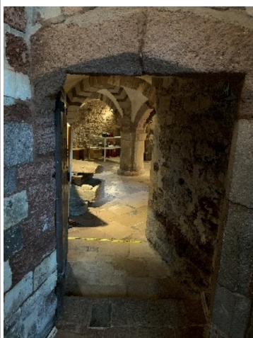
Looking into the Norman cellar
